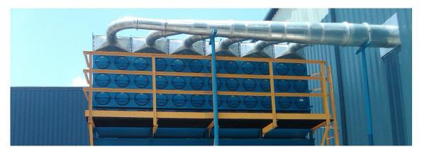
The bulk density and loading of the dust being conveyed is important to consider since these values affect the required conveying velocities in the ductwork. Other considerations include designing elbows/transitions to minimize turbulence and friction, using blast gates to adjust airflow at each pick-up point, and using round ducts over rectangular ones for more uniform conveying velocities.
